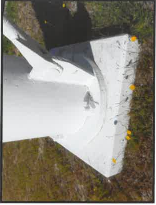
View of the painted concrete foundations and base plates.
